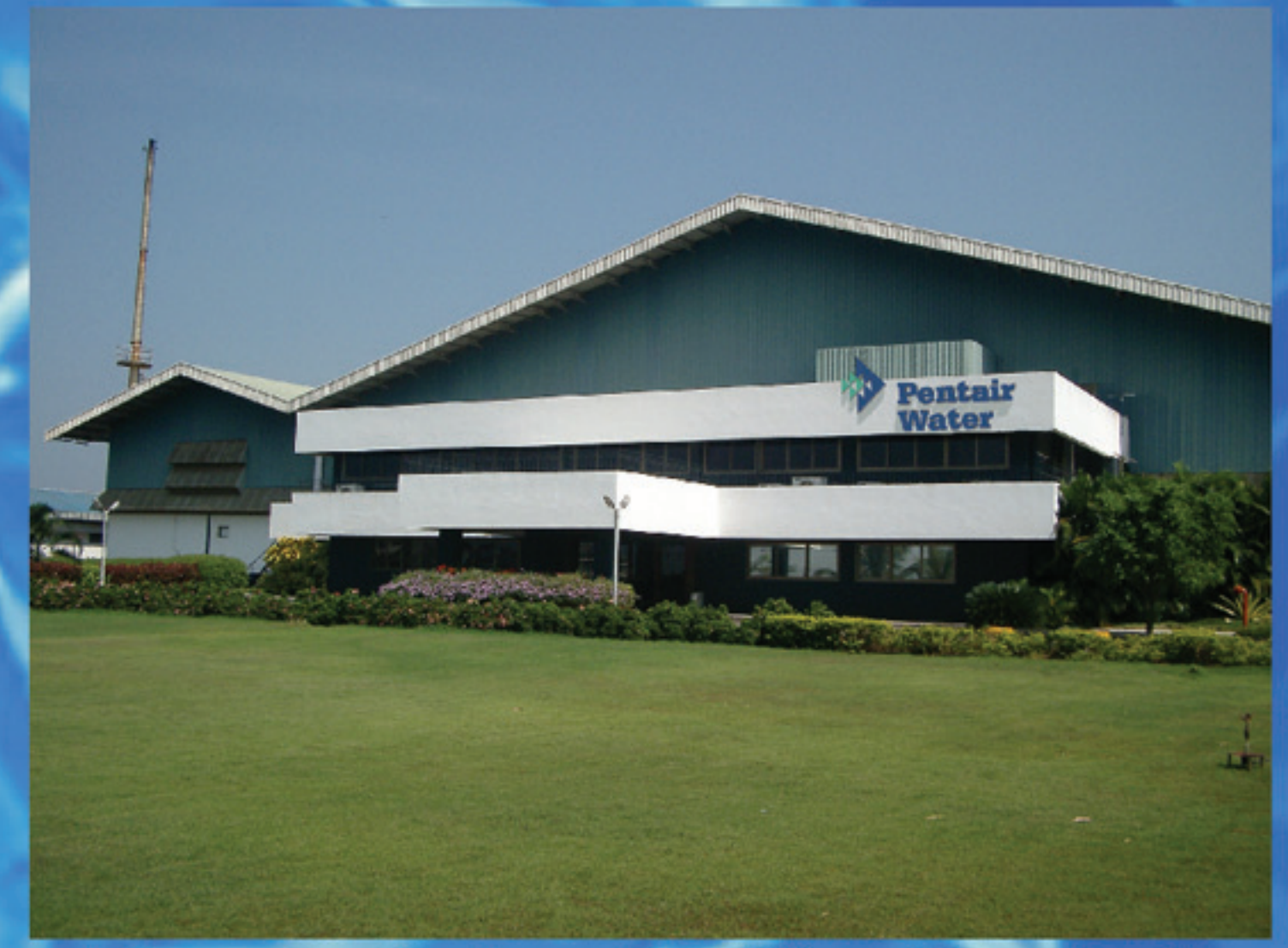
Manufacturing Facility, Goa India
